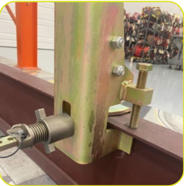
Stanchion installation complete
