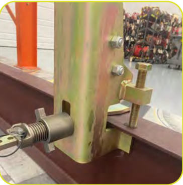
Stanchion installation complete
