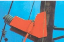
Pole bracket and insulator base cover
