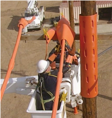
Strong memory improves grip when applied to the utility pole. The pole guard has high impact properties suitable for cold weather service.
