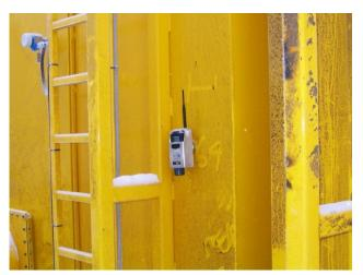
The portability of semi-fixed gas detectors allows treatment facilities to quickly deploy gas detection systems as needed. For example, gas detection systems are needed when facilities must shut down existing process equipment in order to perform routine maintenance.
