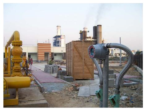
proximity to processes that produce toxic and flammable gases are all potential locations for fixed-head gas detectors.
